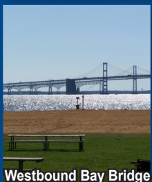
Westbound Bay Bridge
