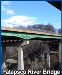
Patapsco River Bridge
