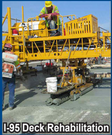
I-95 Deck Rehabilitation
