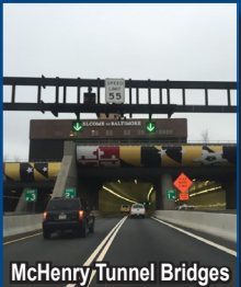
McHenry Tunnel Bridges
